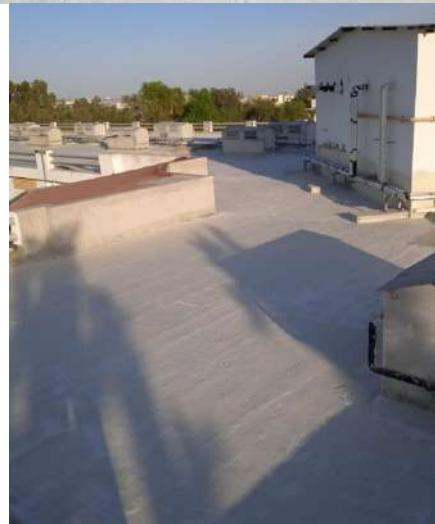
Application and finish product example of the roof insulations
