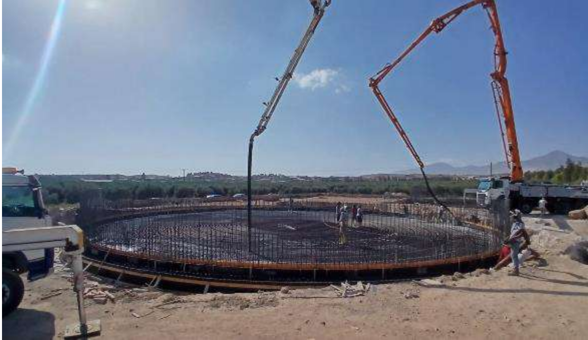
Biogas Project Infrastructure Construction
